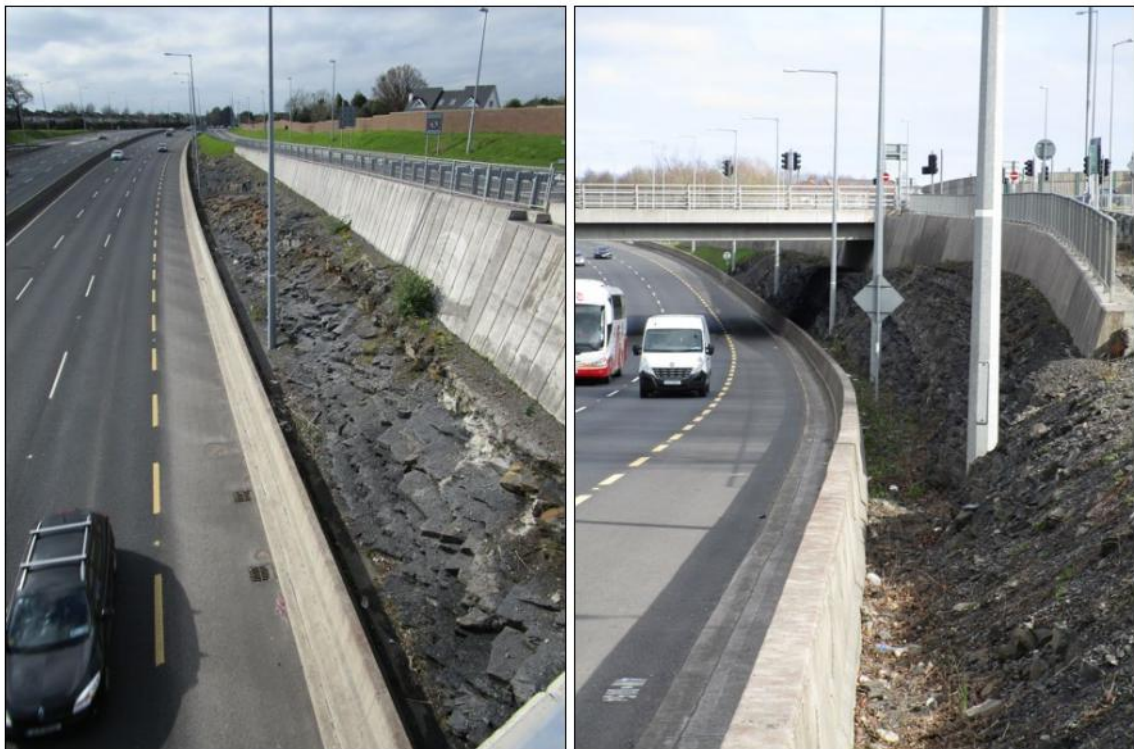
The north west section from the bridge.
