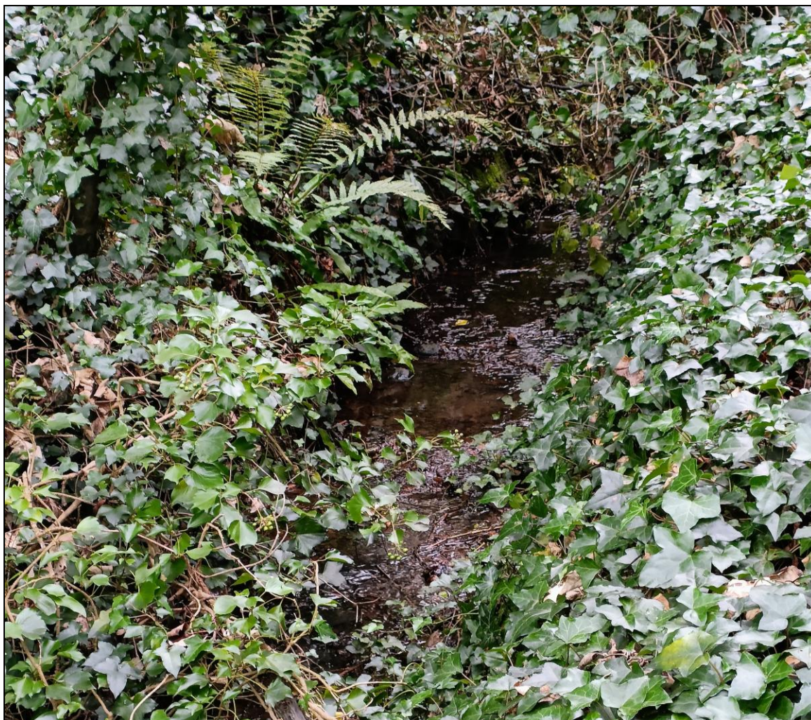
Figure 4-8: A section of the drainage ditch located in the north-east of the site
